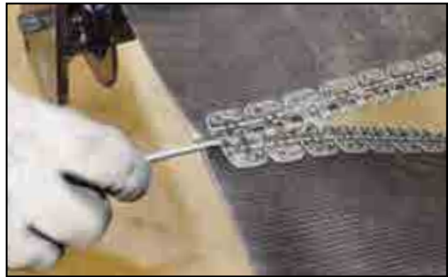
Fig 31 - Thread lacing cable
